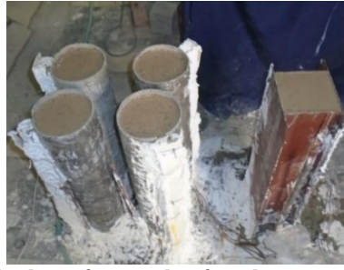
Fig. 5. Filled column formworks after placement and vibration.
