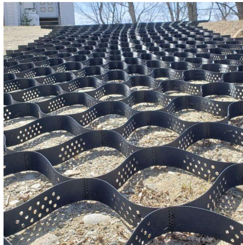
Fig. 1. Geocell reinforcement.
