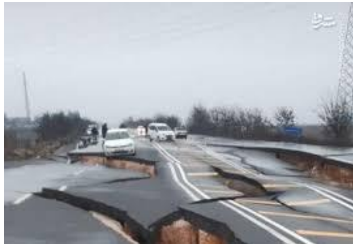
Fig. 5. Vertical cracking in a road embankment during the Haiti earthquake.
