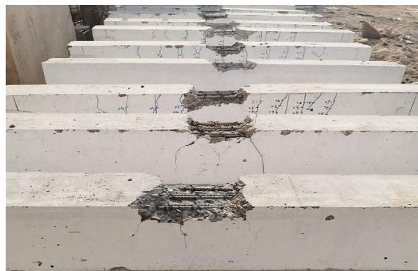
Fig. 2. Damage at the bottom of the specimens (Inverted Specimens).
