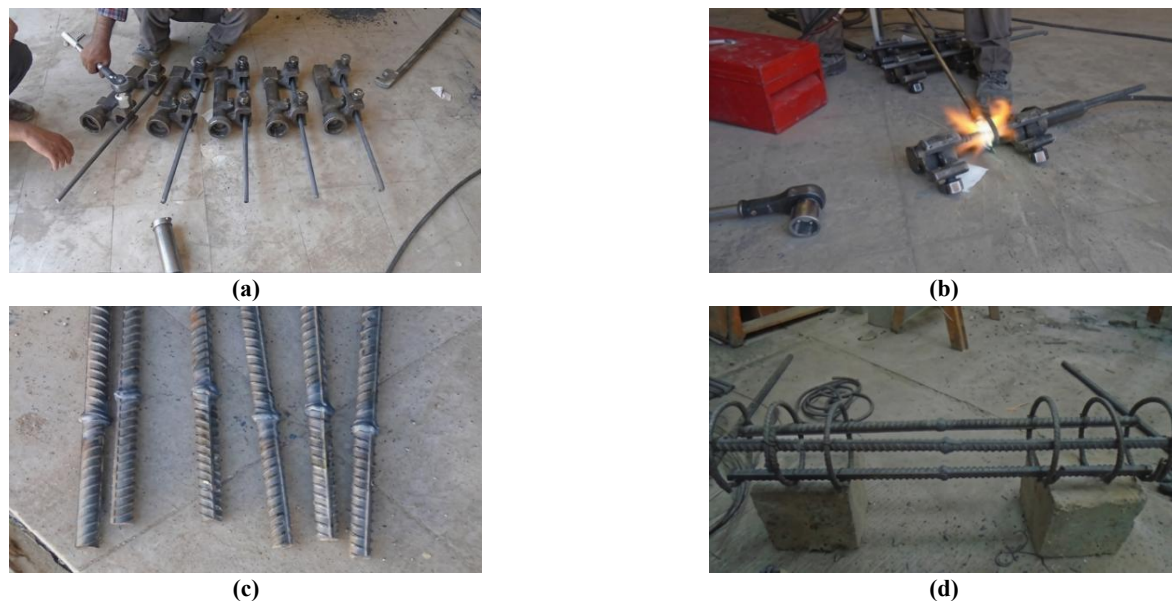
Fig. 4. (a) Longitudinal clamped rebars prior to heating; (b) heating procedure; (c) Rebars spliced by the forging method; and (d) reinforcement cages of the specimens.
